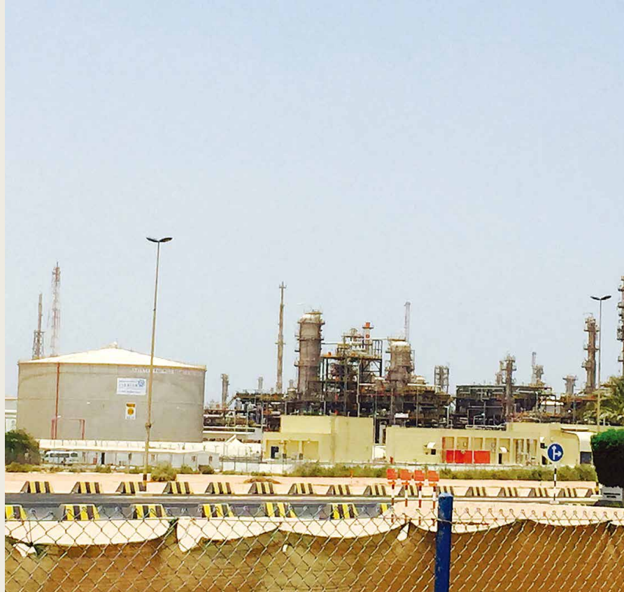
The front view of site
