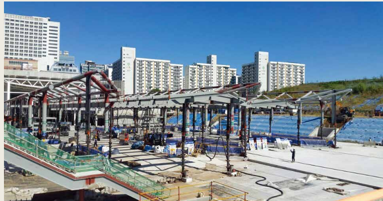
After column cutting 3m and raising
