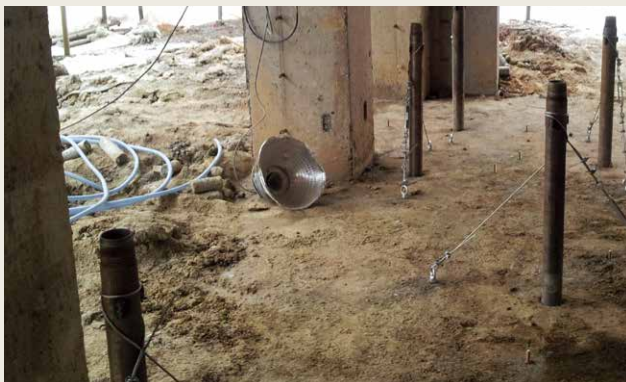
CGS construction method mortar inlet
