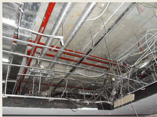
Complicated ceiling of the existing building
