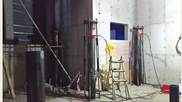
Measuring and pressing piles and pressurizing them simultaneously
