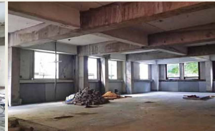
Column removal work was completed
