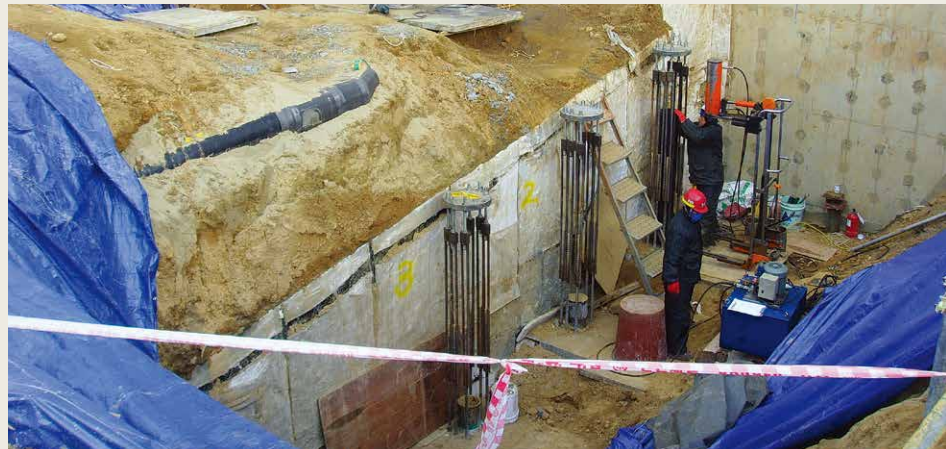
Under construction | top foundation reinforcement, settlement, joint hole, pile, basement reinforcement
