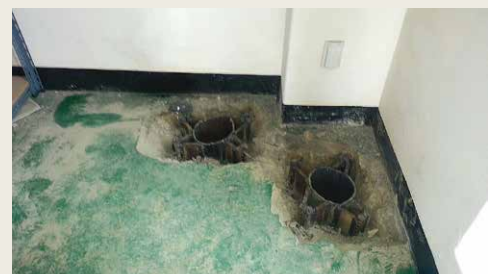
Pressed pile installation-hiding at the foundation
