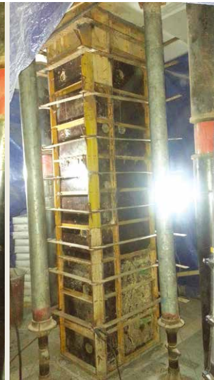
Mold/ placing preparation
