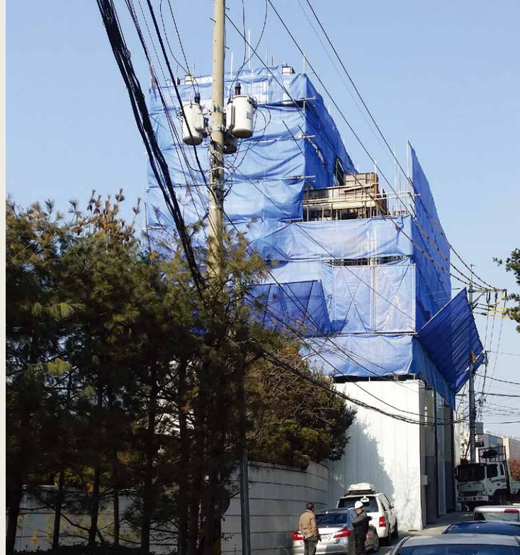
New construction underway on a sloped embankment
