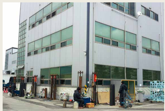
External work of the building
