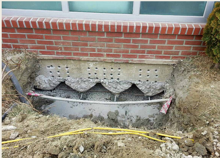
After construction | The settlement was accelerated due to the increase of the weight despite the foundation reinforcement by using top on the soft ground.
