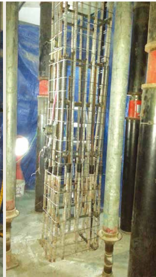
Column steel bar reinforcement/ binding
