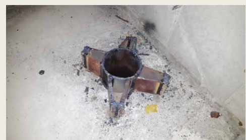
Pressed pile installation-exposure on the foundation
