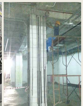
Wire rope binding column reinforcement
