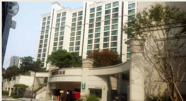
After remodeling of elevator underground extension
