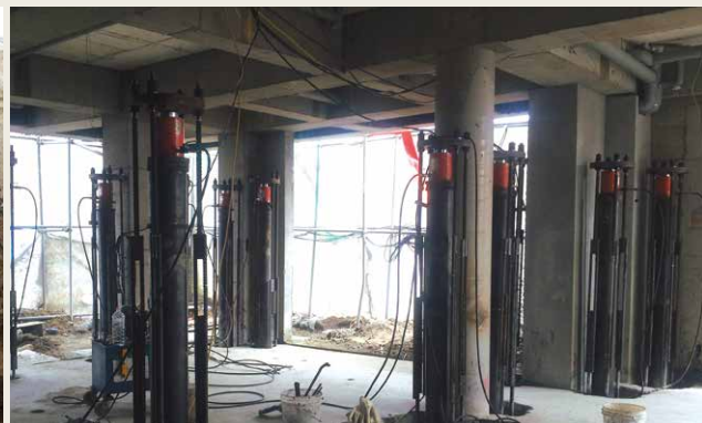
Under construction of pressing piles
