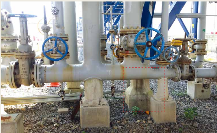
Column foundation reinforcement within dotted line
