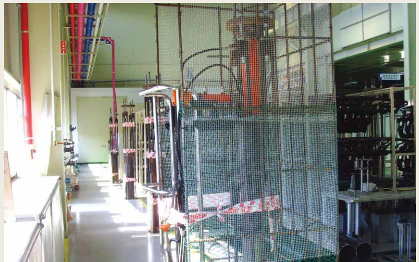
The first construction | foundation reinforcement reconstruction
