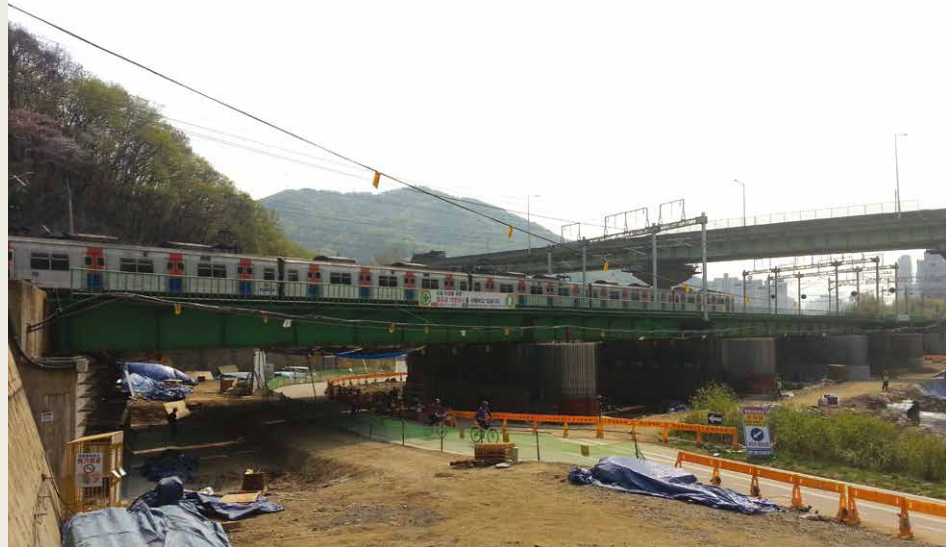
The front view of Anyangcheon Stream railroad bridge
