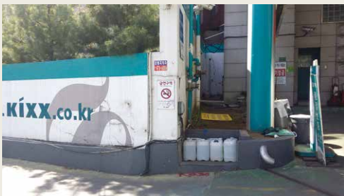
Existing retaining wall
