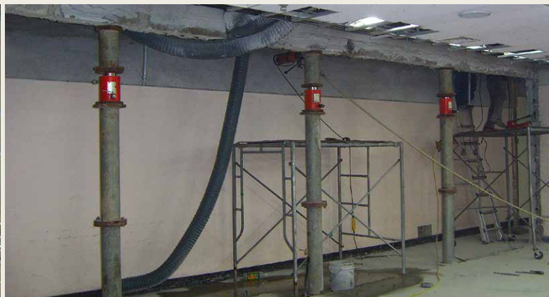
Under construction | removal by supporting as Jack-up pile
