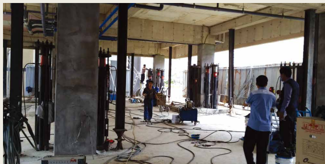
Under punching reinforcement and reconstruction
