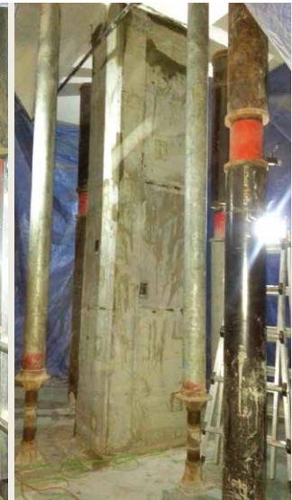
After placing/ reinforcement completion
