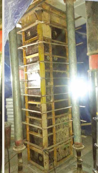
Mold/ placing preparation
