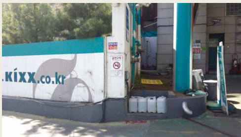
Existing retaining wall
