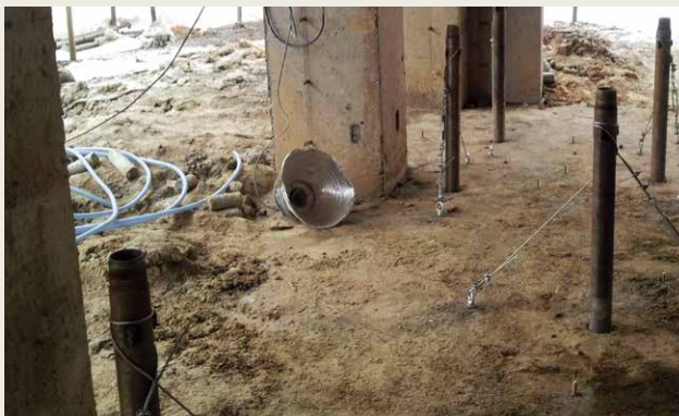
CGS construction method mortar inlet
