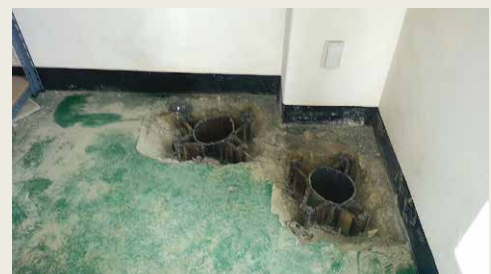
Pressed pile installation-hiding at the foundation
