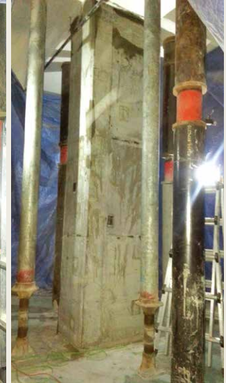
After placing/ reinforcement completion
