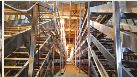
Underground joint hole was completed after connecting the underground tunnel connection
