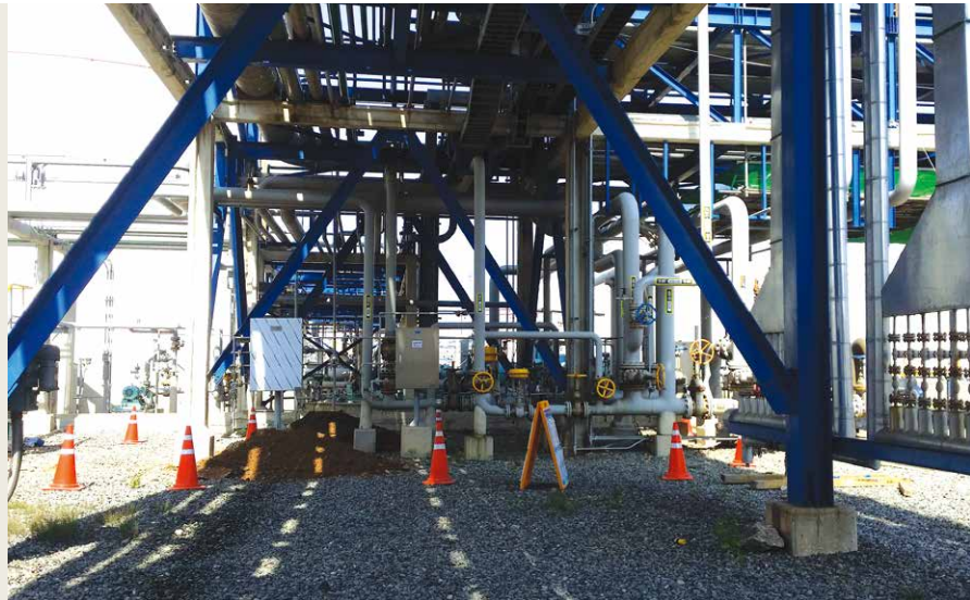
Current status of Pipe Rack Foundation reinforcement location
