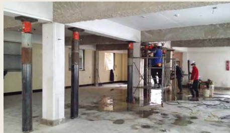
Column removal work by using Jack-up
