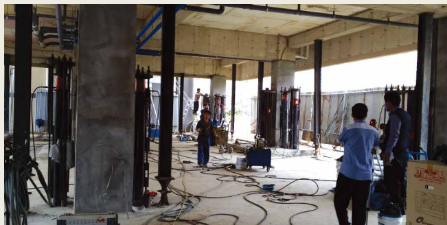
Under punching reinforcement and reconstruction
