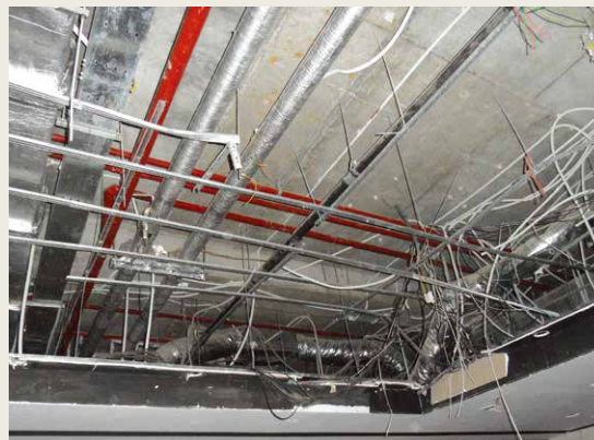
Complicated ceiling of the existing building
