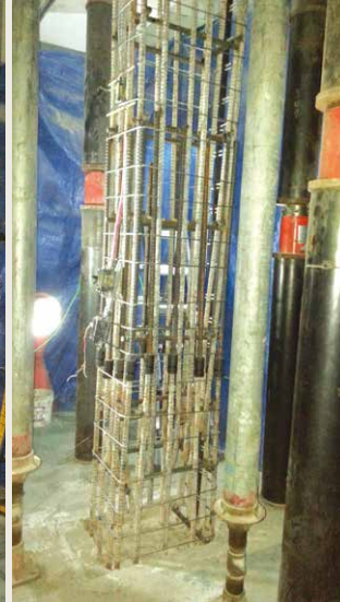
Column steel bar reinforcement/ binding
