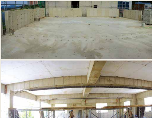
After construction | Slab top and bottom
