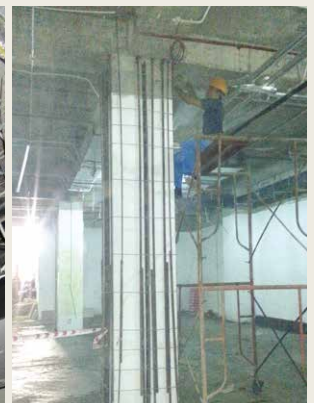
Wire rope binding column reinforcement
