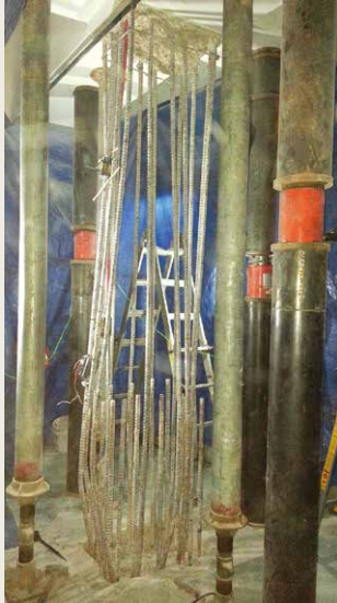
Vertical steel bar buckling
